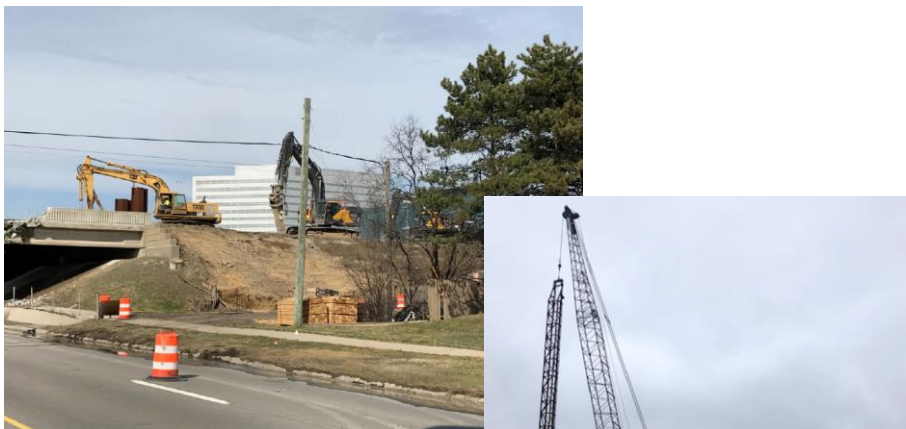
Livernois Bridge Demolition
