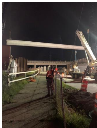
Bridge Beam setting at Coolidge Hwy
