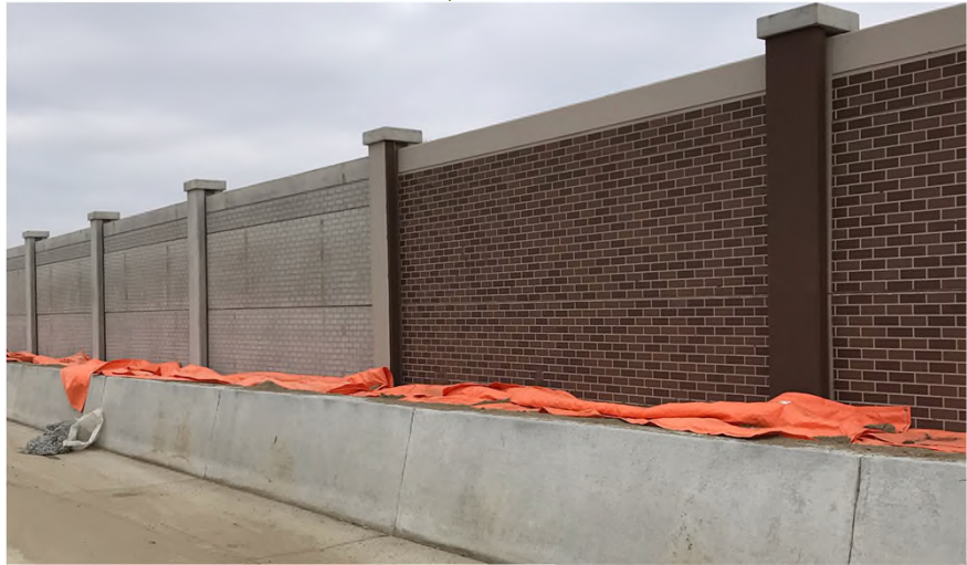
Sound Wall Construction
