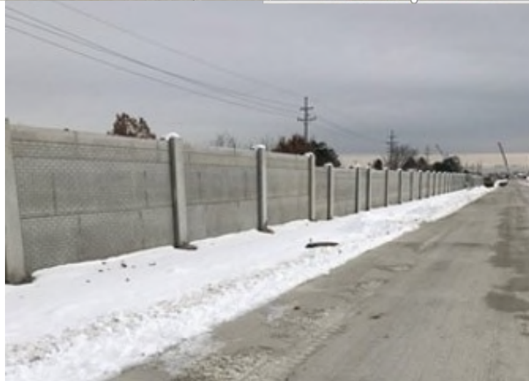
Sound Wall Completed Aesthetics/Painting To Be Completed Next Year
